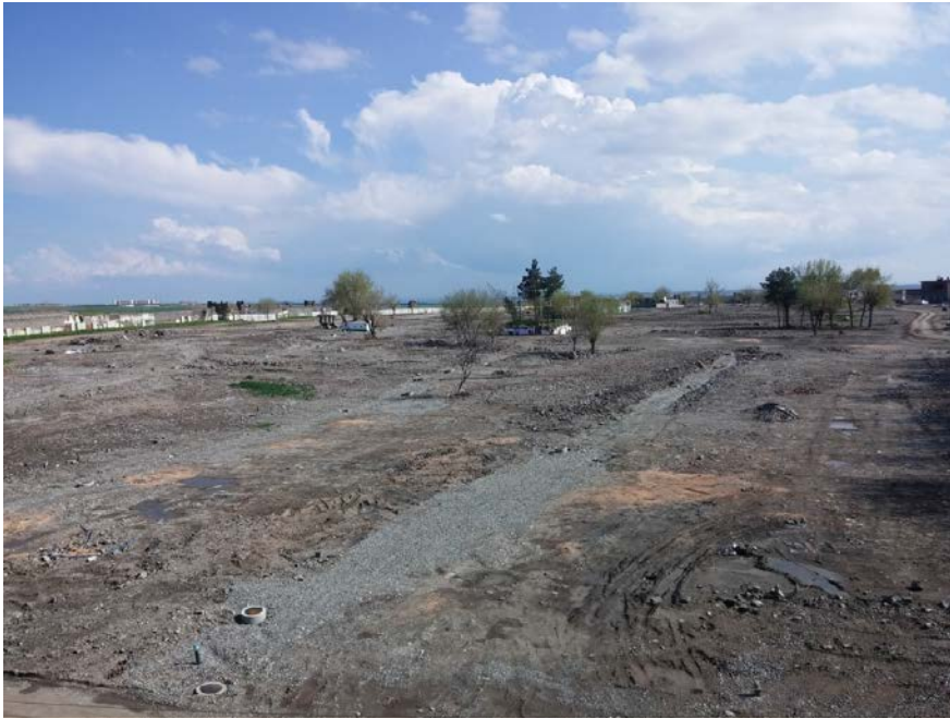
Picture taken from a commercial flight 4 May 2017 showing ongoing destruction
